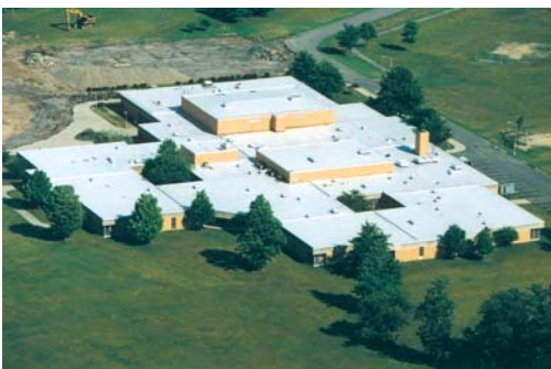
Schools in northern climates as well as in the south enjoy Flex benefits for saving air conditioning energy costs.
