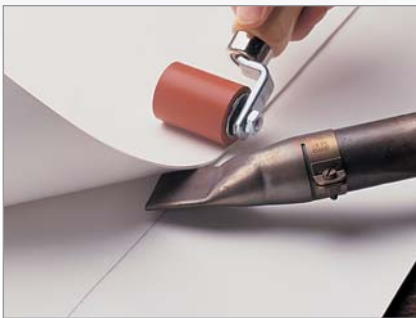
Hot-air welded Flex seams are as strong as the membrane itself.
