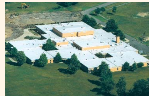
Schools in northern climates as well as in the south enjoy Flex benefits for saving air conditioning energy costs.
