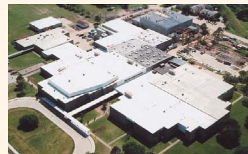
Flex Cool Roof systems offer measurable benefits for energy saving: Solar Reflectance .87 Thermal Emittance .90
