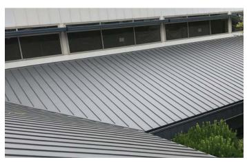
The product's base flange is approximately 2" wide and the rib profile is 1-1/8" high. Each rib has an 1/8" diameter fiberglass reinforcing cord built in for dimensional stability.
