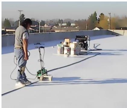
**2** The membrane is laid into position and membrane seams are hot air welded.
