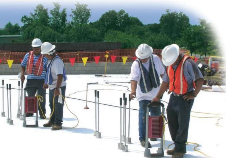
**The new Flex RhinoBond high-production attachment technique is fast and easy on workers, and provides superior uplift resistance.**
