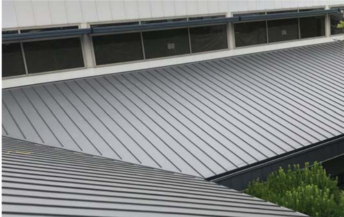
The product's base flange is approximately 2" wide and the rib profile is 1-1/8" high. Each rib has an 1/8" diameter fiberglass reinforcing cord built in for dimensional stability.
