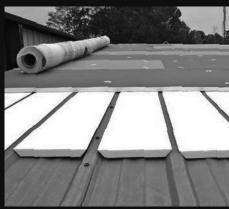
Flex RhinoBond is also an ideal option for metal roof retrofit applications. Because the system does not require in-seam fastening, the membrane seams do not have to be positioned over the purlins. This eliminates the need for specialty purlin-width sheets, simplifies the installation and reduces waste.
